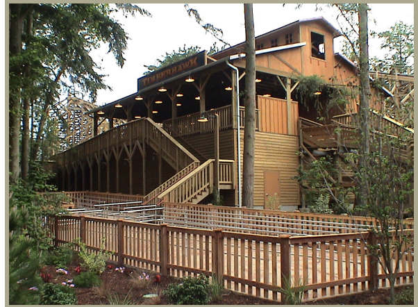
Coaster station with que area (foreground), stairs to 15-ft high loading & unloading deck, and coaster exit track (at right).
