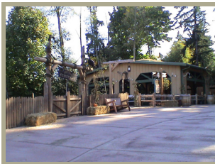
Dodge'ns is a relocated steel canopy themed in wood construction.
