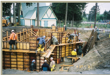
Forming the Timber Axe foundation
