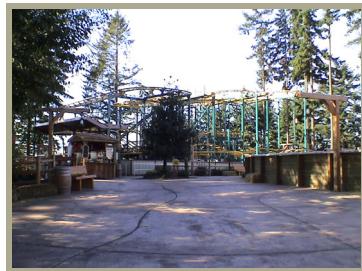
Rides, Kiosks and Concrete Flatwork
