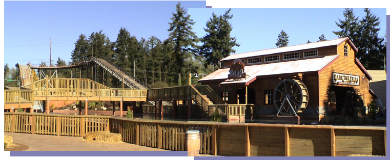
Lumberjack Falls was constructed while the park was open.
