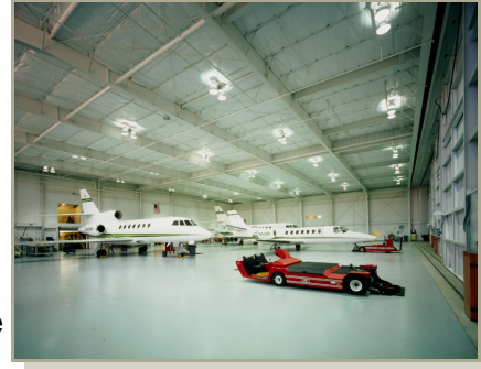
The 20,000 sf hangar features in-floor heat.
