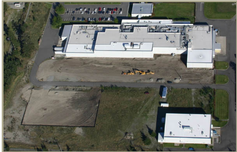
Toray Composites site showing graded pads for expansion in foreground
