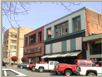
Broadway elevation prior to renovation
