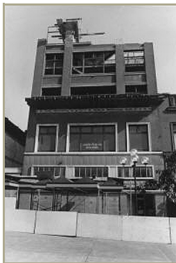
1976 photo of top floors of the New York building being demolished.
