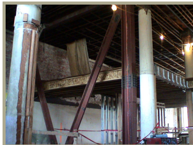
New structural steel and floor framing adjacent to original columns.
